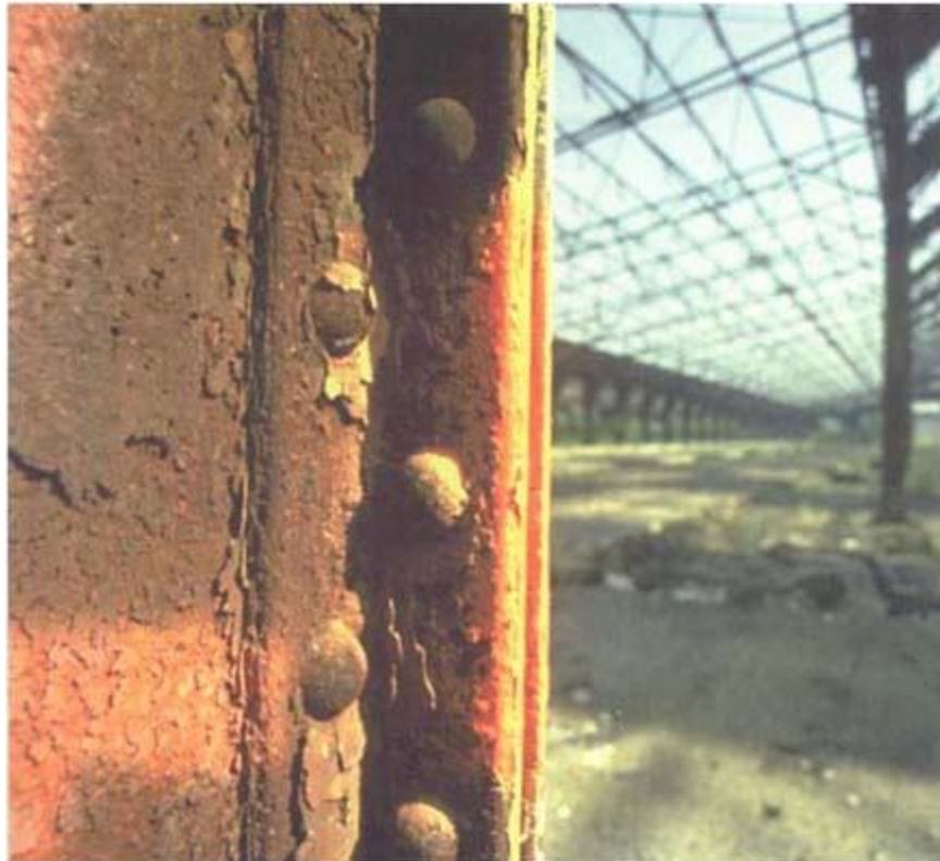
*Rust covers a steel beam of an old train station.*
